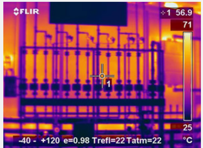
Fig. 2: Picture made with a thermographic camera
